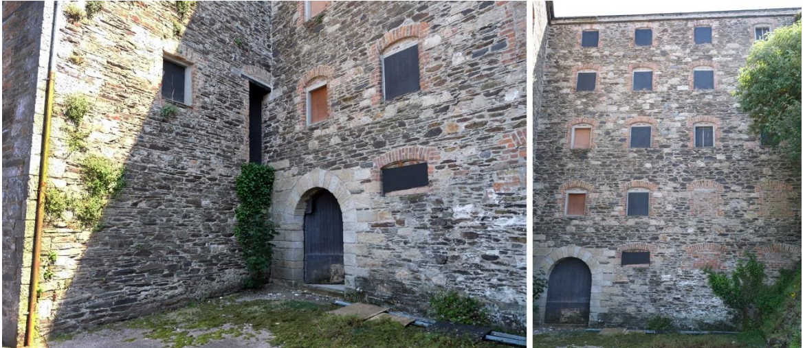
Fig.23: View of the junction between the north elevation and the offset return showing a granite ashlar doorway at ground floor level, with brick windows and rubble masonry mirroring that seen elsewhere on the building.
