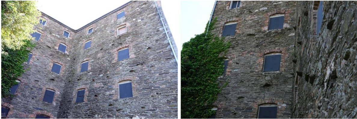
Fig.19: The north elevation of the off-set return and adjacent west elevation of the main building is again composed of random rubble masonry punctuated by brick window openings, but with projecting rough stone corbels arranged in a diagonal pattern (probably to support chutes) which are a distinctive feature of the elevation.
