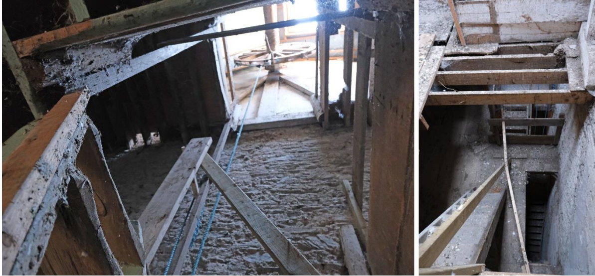
Fig.28: View of the winch shaft (left) and internal staircase (right).
