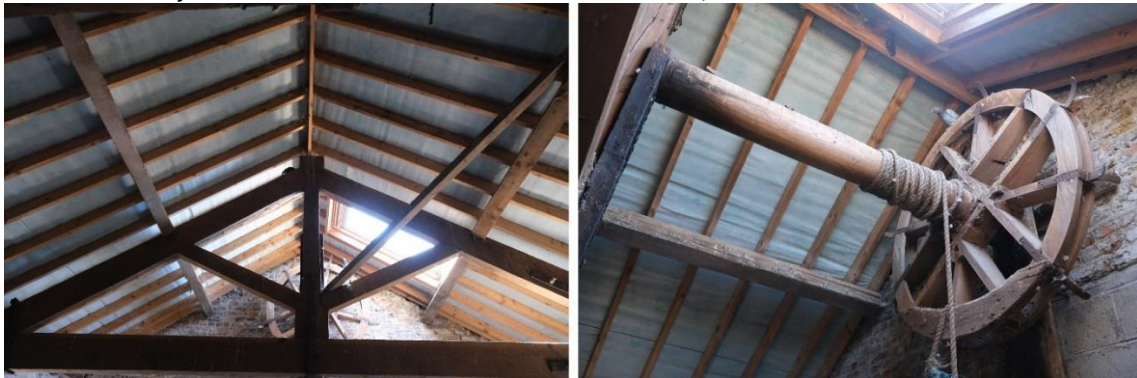
Fig.26: Detail showing replacement roof cover (left) and winch.
