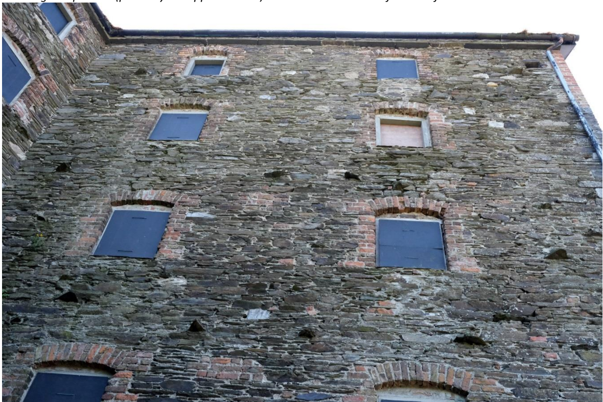
Fig.20: North elevation of the off-set return showing projecting rough corbels.
