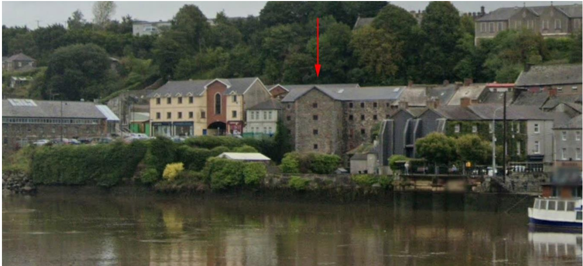
Fig.32: View of the grain store from the bridge. The external lift will be visible. The café/restaurant will be marginally visible.
