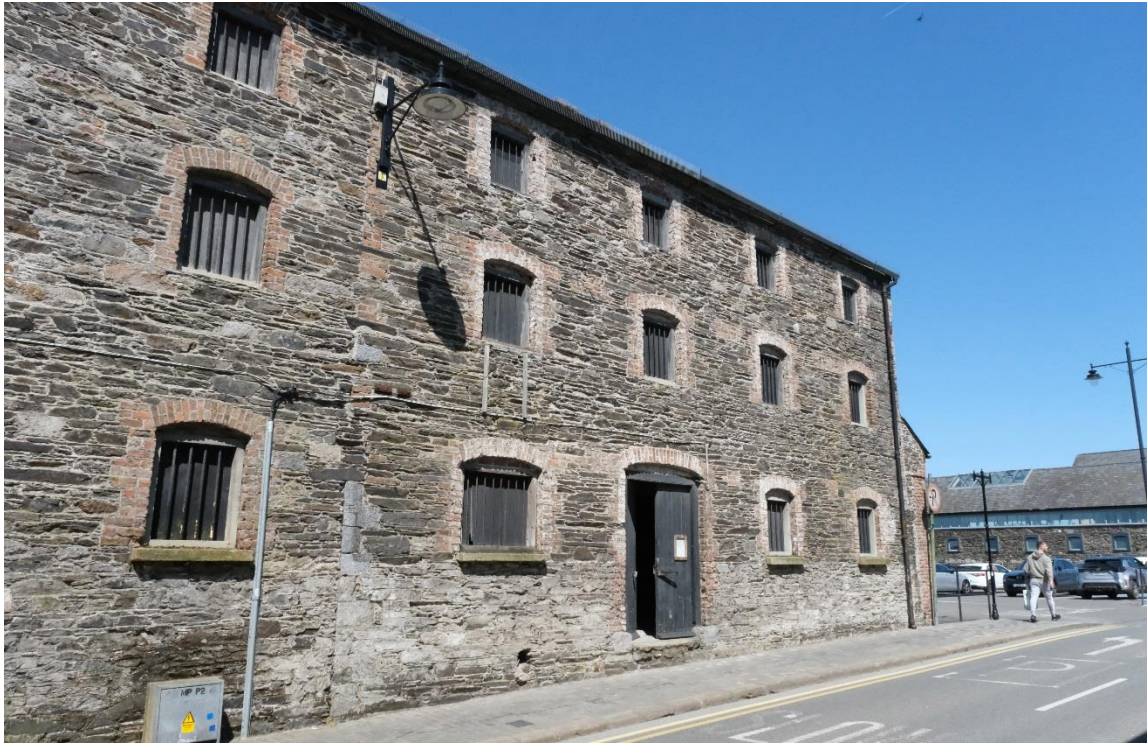
Fig.14: View of the northern part of the façade showing limestone quoins at ground floor level marking the separation between the two buildings, with matching treatment of masonry and detail in both parts.
