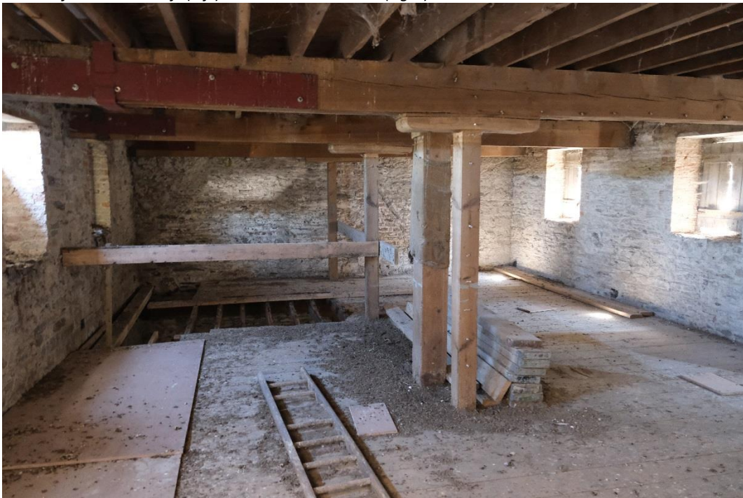
Fig.29: The interior is plain and unfurnished without wall or ceiling finishes, with plain rubble walls and window reveals throughout, sometimes retaining timber shutters.
